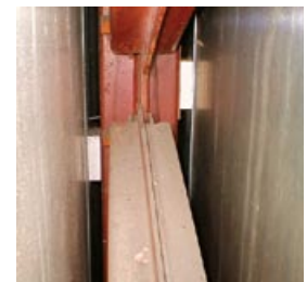
Figure 22 AIB offcuts used as packers around column in CLASP building
