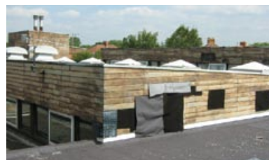
Figure 23 AIB fascia panels with wood effect finish
