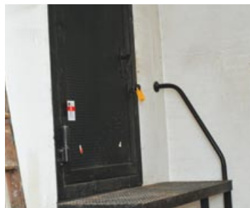
Figure 45 'Durasteel' composite steel and asbestos fire door
