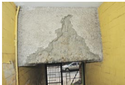
Figure 8 Sprayed coating on building passageway
