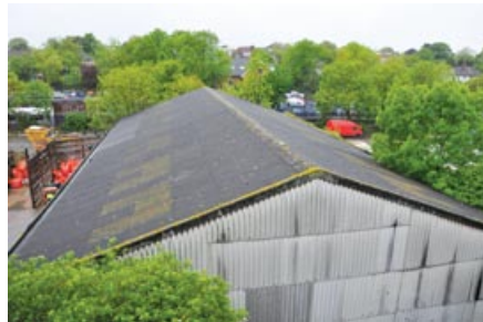
Figure 32 Asbestos cement roof and cladding
