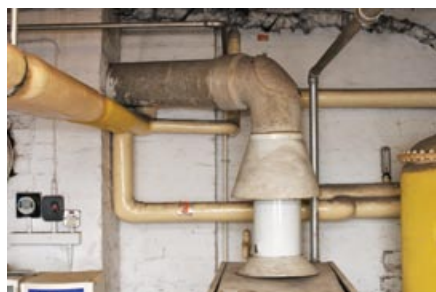
Figure 34 Asbestos cement boiler flue
